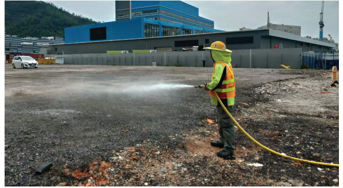
灑水防塵 Dust Control
