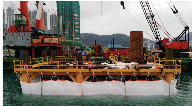
隔泥幕 Silt Curtain
