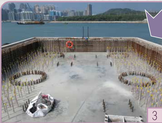
部份完工的樁帽 Partially completed pile cap
