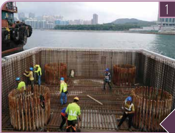
於樁帽殼內扎鐵 Reinforcement bars are fixed inside pile-cap shell
