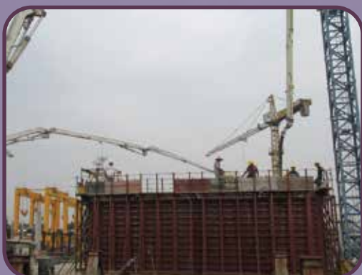
灌注混凝土 Placing concrete
