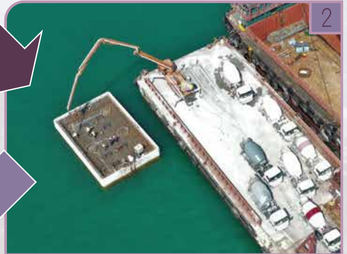
澆灌混凝土 Placing concrete for pile cap
