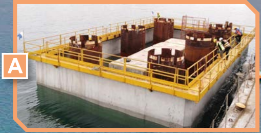
A 已安裝樁帽殼 Pile-cap shells installed
