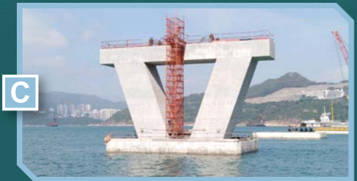
C 已安裝預製V型橋墩 Precast V-pier installed
