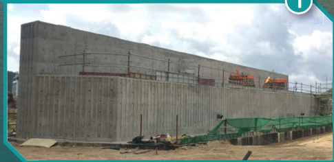
興建橋台 Construction of abutment
