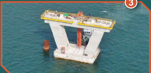
安裝V型橋墩 Erection of V-pier
