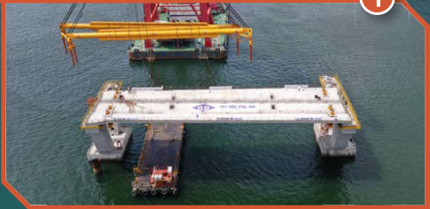
安裝預製箱形橋樑 Erection of precast box girder
