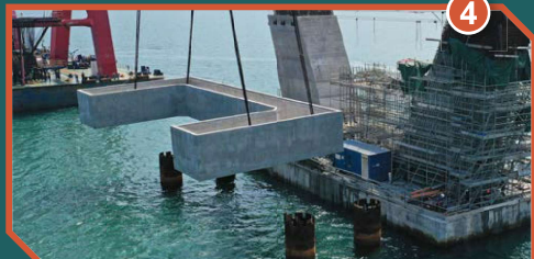
安裝樁帽殼 Installation of pile-cap shell
